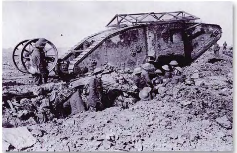
Tanks ▲ Tanks, like the early British model shown above, enabled armies to travel over uneven ground and barbed wire. Although too slow to be used to full advantage at first, they were devastating against soldiers in trenches.
